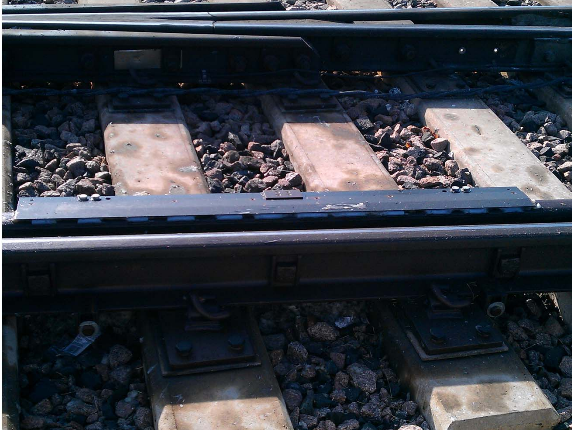
Top of restraining rail applicator bar
