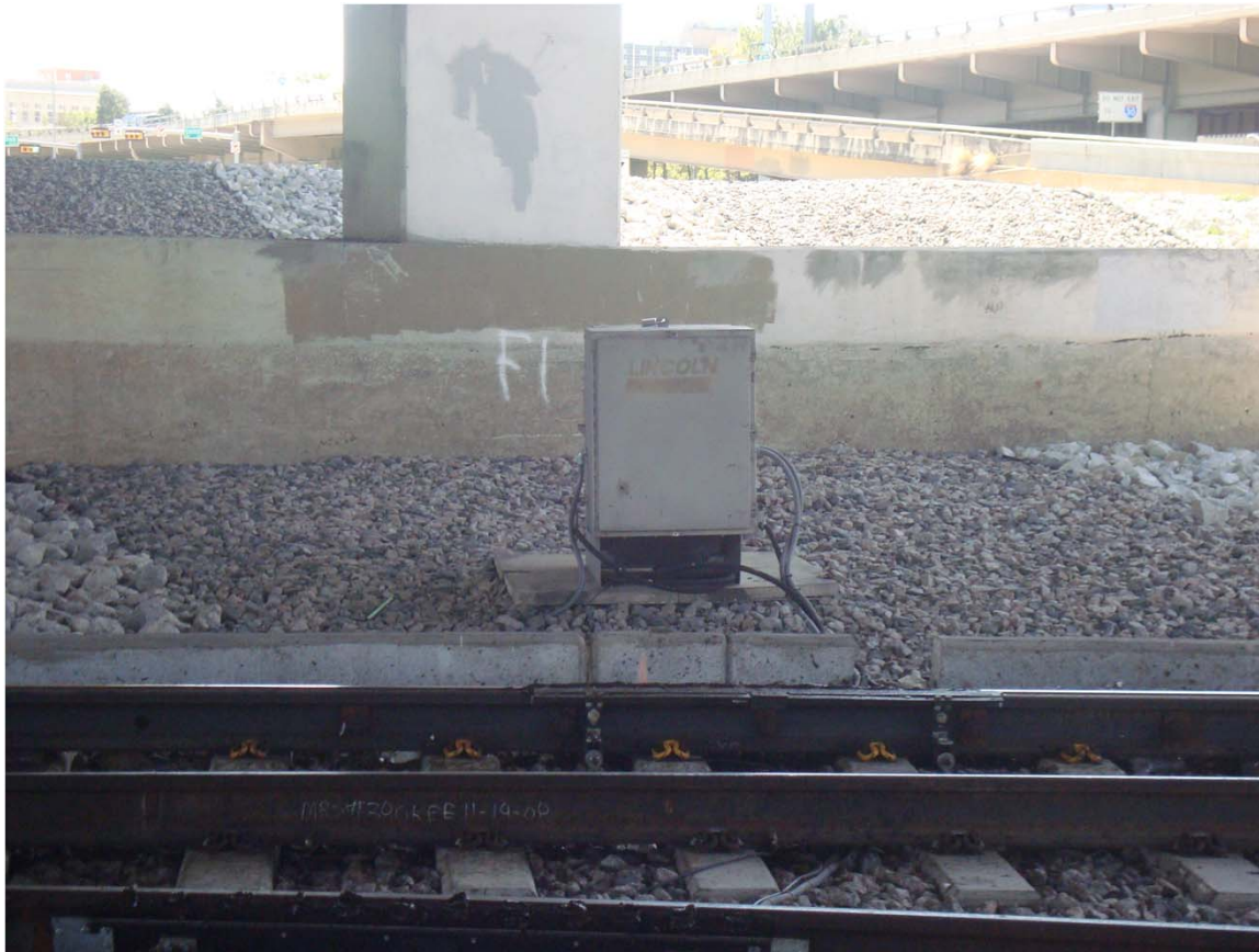
120v Dual pump applicator supplying lube to four track brush bars and two top of rail bars
