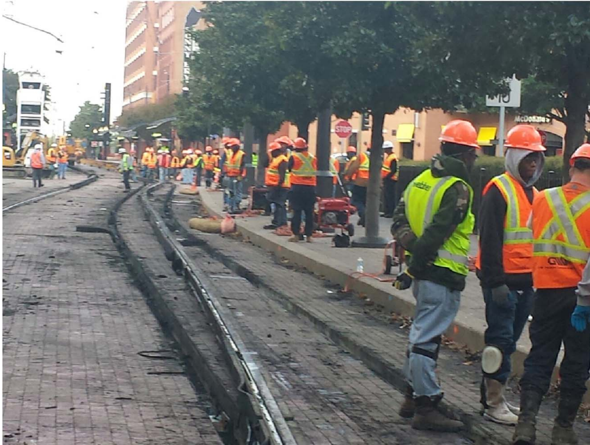
118 lb girder rail being removed
