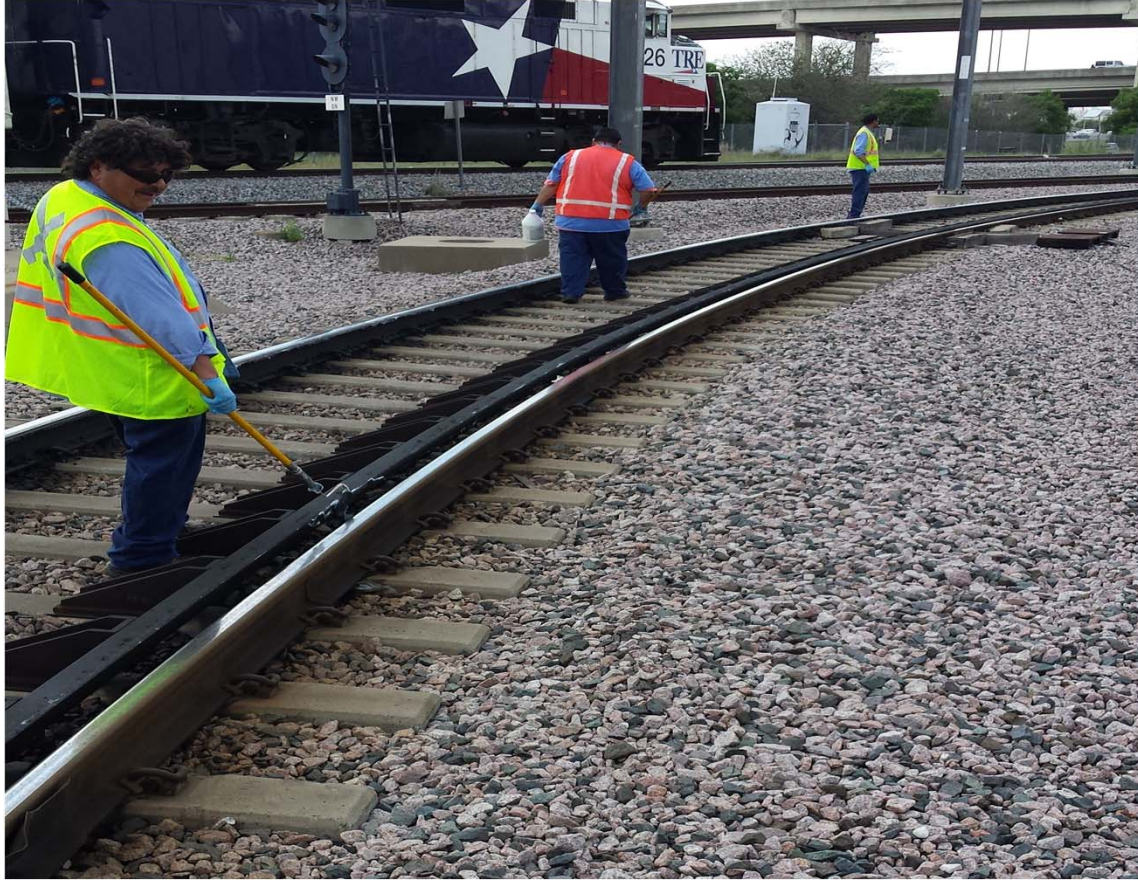
Crew manually applying lubrication
