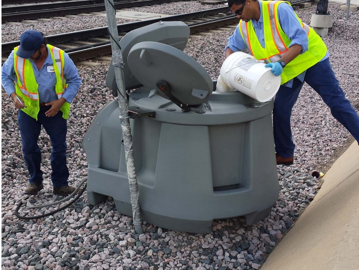
Crew filling lubricator unit
