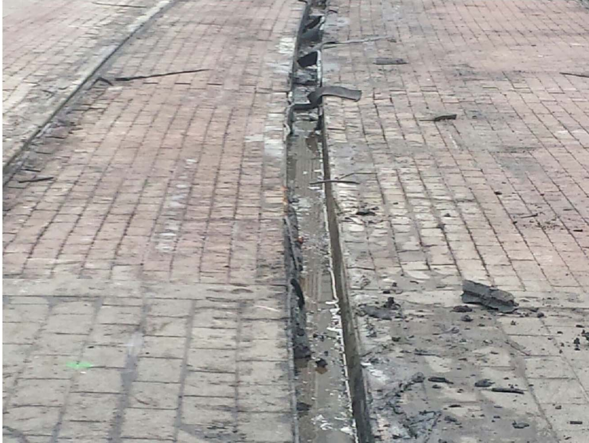
118 lb girder rail being removed
